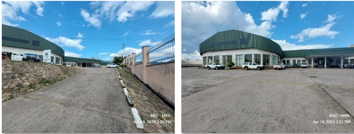
Figure 2-1. The existing office building showing its entrance and exterior area
